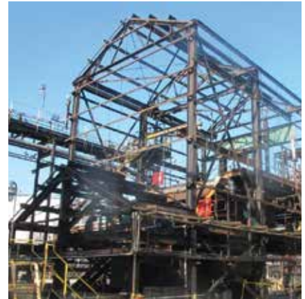
This portion of the former Koppers plant underwent precleaning and abatement.
